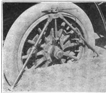
Fig. 3—A handy and powerful jack for mud runs
